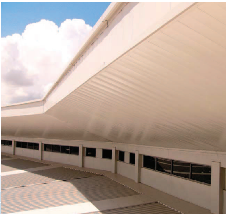
Industrial Factory, Singapore
