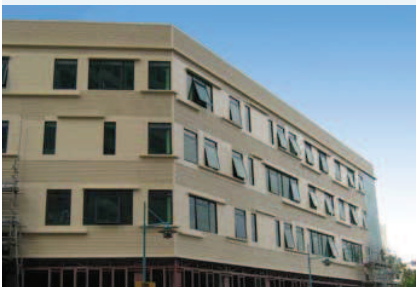
Tan Tock Seng Hospital (Extension Building)
