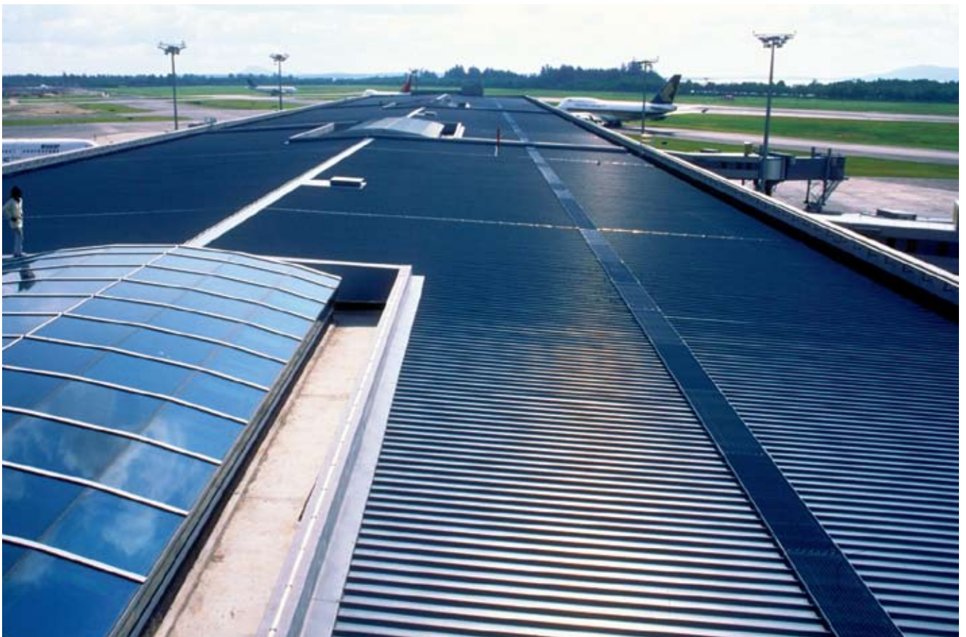
Changi International Airport, Terminal 2
